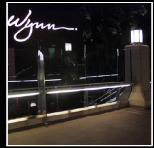
Pedestrian Bridge, Las Vegas, NV
